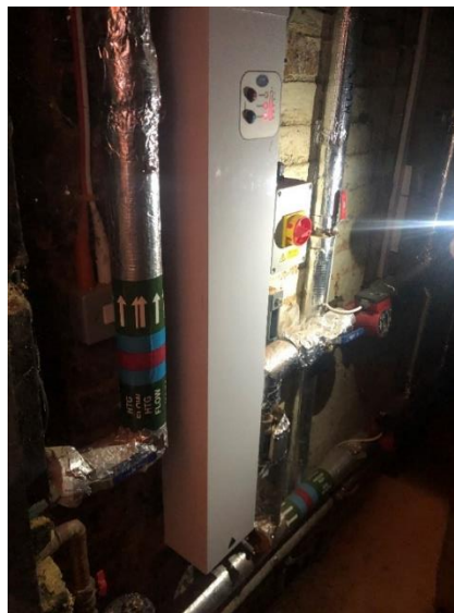
Figure 30 – Inline Backup/Top-up direct electric heater
