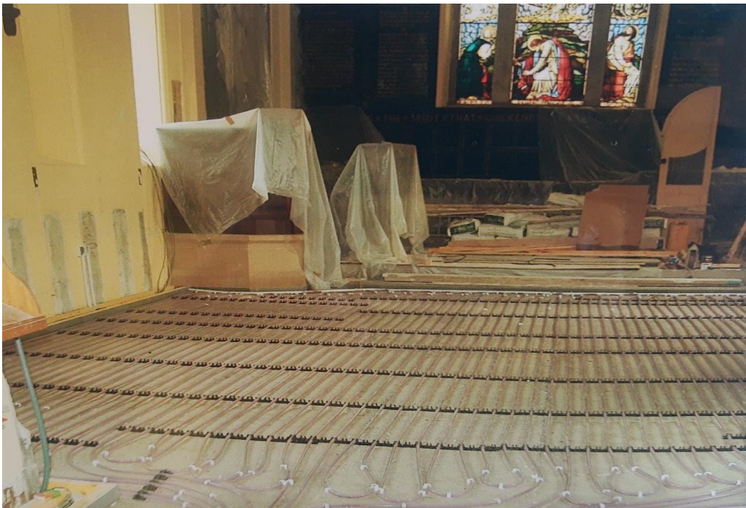
Figure 18: UFH pipework being laid down during refurbishment works
